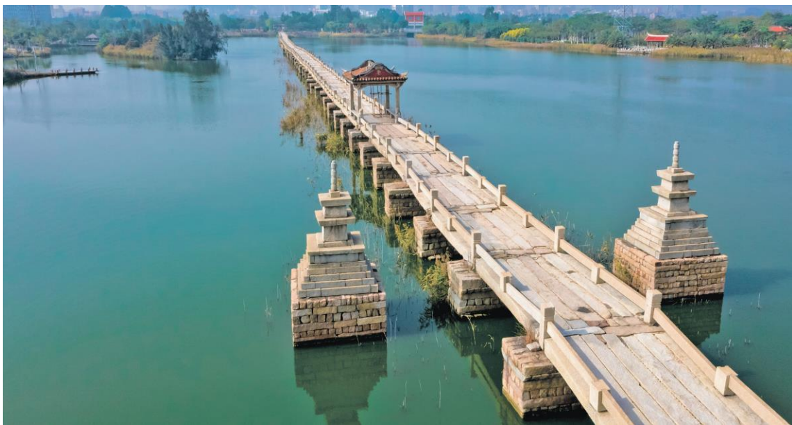
Anping Bridge, one of Quanzhou's important transport links.
